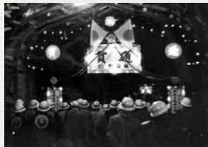
In February 1958, the most difficult part of the Kurobegawa No. 4 project, the Kanden Tunnel, was completed.
