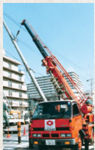
Recovery work after the Hanshin-Awaji Earthquake
