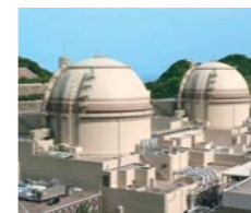
● Ohi Power Plant
