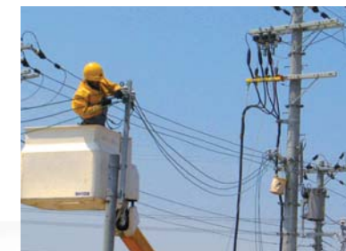
●Distribution line maintenance
