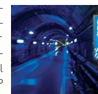
● Kanden Tunnel, which runs through a fracture zone
