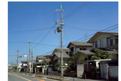
●Electrical pole and transformer
