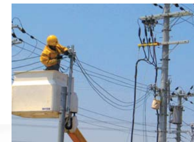
●Distribution line maintenance
