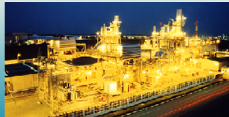
Thailand's Rojana Power Co., Ltd.
