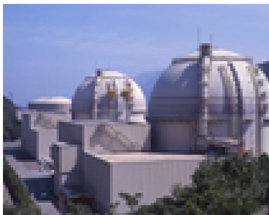
Ohi Nuclear Plant (4,710 MW)
