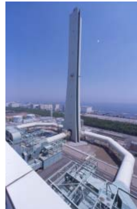
Nanko Thermal Power Plant
