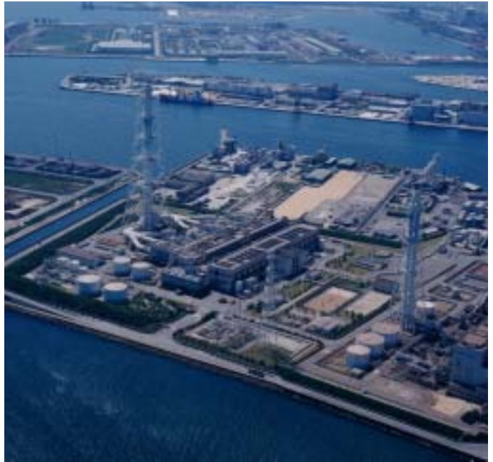
Himeji No. 1 Thermal Power Plant
