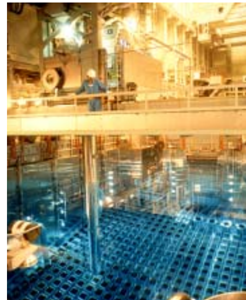
Periodic fuel rod inspection (Takahama Nuclear Plant)
