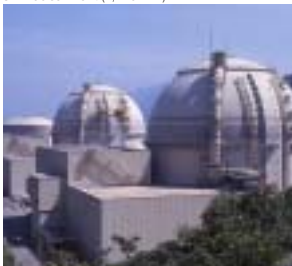
Ohmi Nuclear Plant (4,710 MW)
