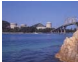
Mihama Nuclear Plant (1,666 MW)
