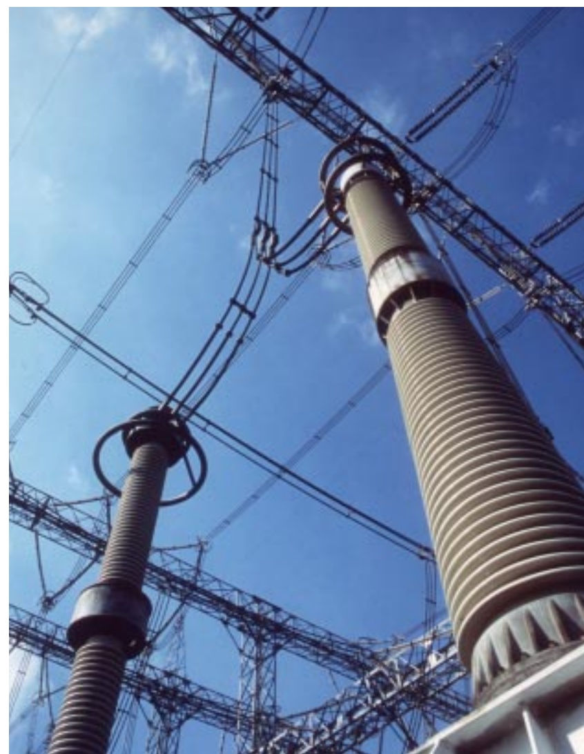
(from top) Transmission network map Shin-Ikoma Substation
