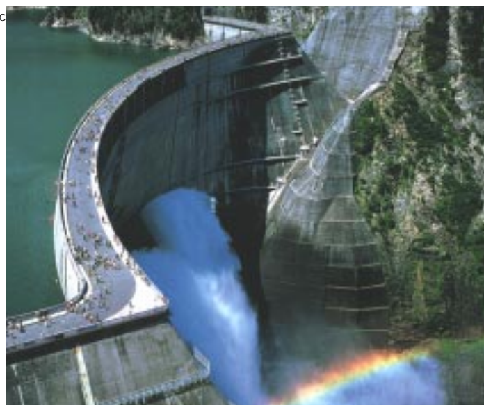
Kurobegawa No.4 Thermal Power Plant (335 MW)
