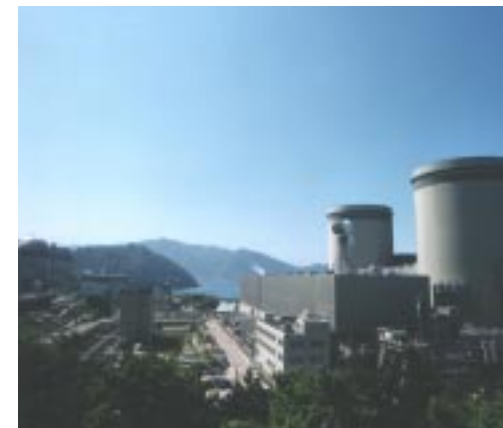
Nuclear power plants (from left): Ohi Plant (4,710 MW), Mihama Plant (1,666 MW), Takahama Plant (3,392 MW)
